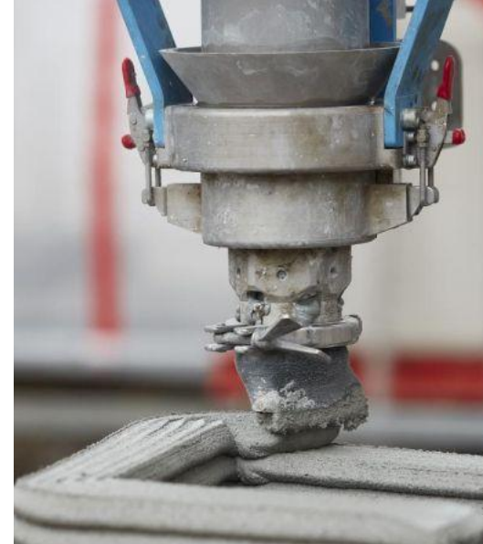
3D concrete printing
